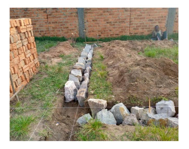
Mortar being placed between foundation rocks. Note pan for mortar in the back behind the bricks.
