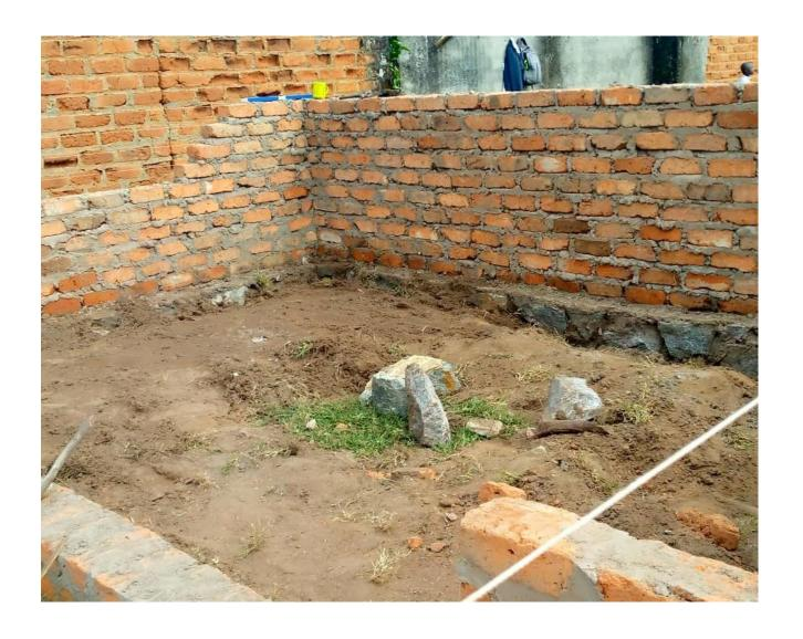
Brick walls being placed on top of foundation.
