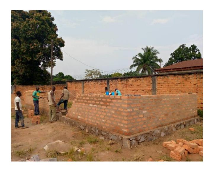
Brick walls being placed on top of foundation.
