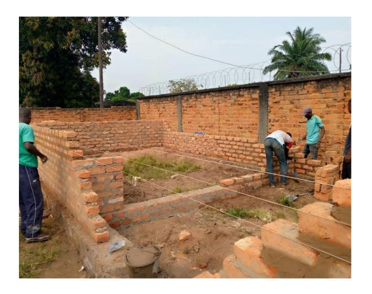
Closer view of brick walls being placed on top of foundation.
